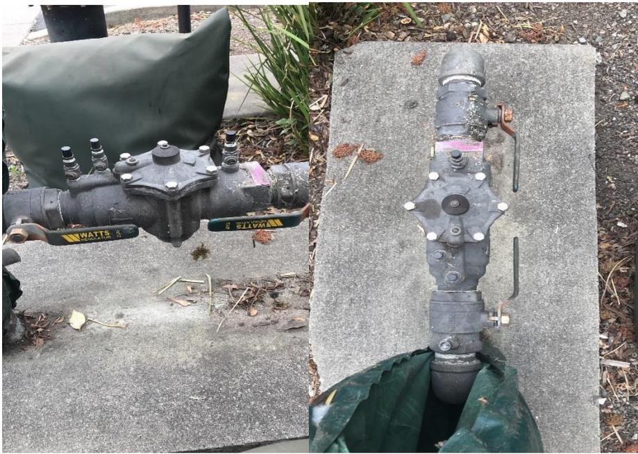
There are also "low hazards" such as a well on a property, a property with pumps, or a property with a residential fire sprinkler system. Properties with low hazards are required by State Health Code Title 17 to have a double check (DC) backflow device. The double check backflow device is a valve with two independent check valves that are spring loaded that allow water to flow through the device to the property but prevent water from flowing back.
