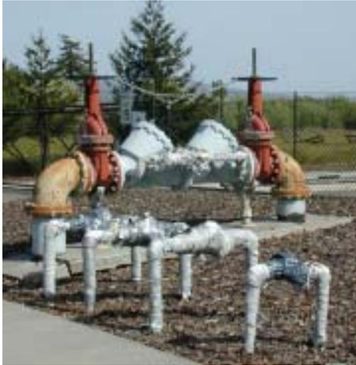
*Fig. 1.3.12 Backflow preventers are often prominently placed at building entries. Consider alternative placement and screening of devices.*
