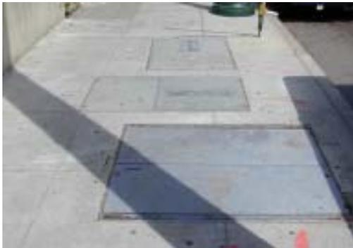
*Fig. 1.3.13 In downtown settings, meters are commonly placed in vaults or boxes below grade. Consideration should be given to this approach in other locations.*
