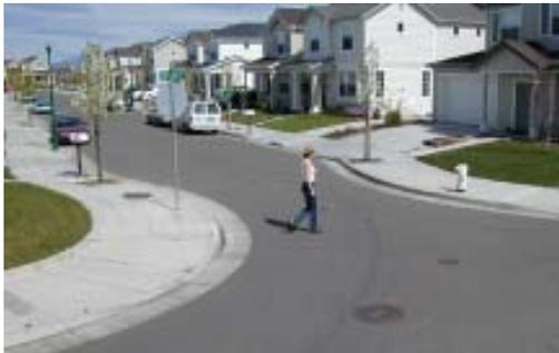
Fig. 1.1.10 This 30 foot street with a neck down slows traffic and shortens the crossing distance.
