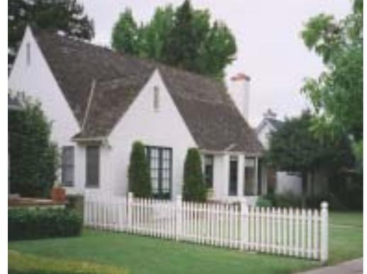
Fig. 4.7.11 Picket fence with 36 inch posts and 30 inch pickets.
