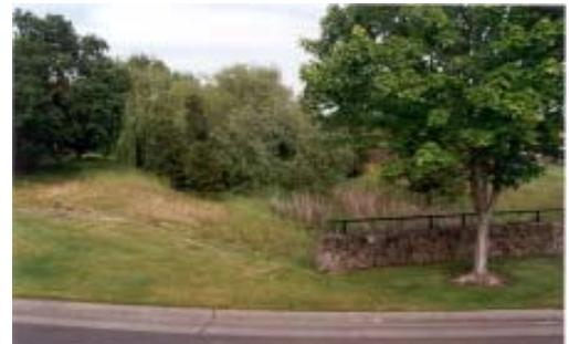
Fig. 4.4.8 The Countryside development of Fulton and Hall Road incorporates a large natural swale for storm drainwater as opposed to putting it in a pipe.
