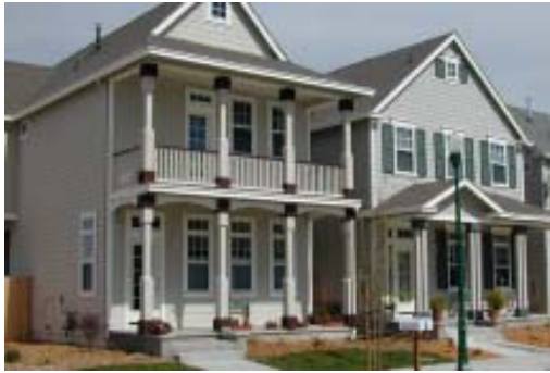
Fig. 3.1.7 These homes which are served by an alley create a streetscape without garages.
