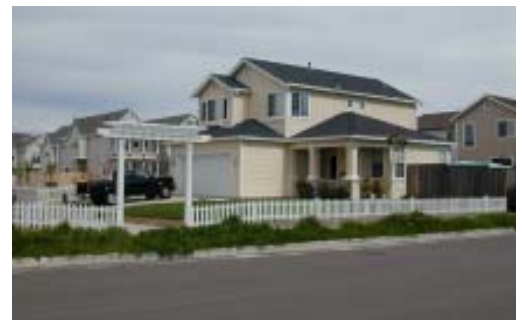
Fig. 3.1.6 Front-on or side-on treatment is preferred to back-on. This side-on treatment permits pedestrian and bike access and creates a more pleasing streetscape.
