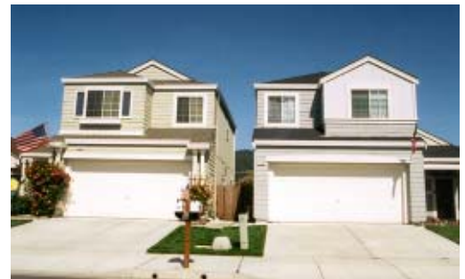
Fig. 3.1.22 This subdivision has several problems. The garage doors are too dominant. The front door and the living spaces are too far from the street. Although there was some effort made to vary the roof forms, the homes are too repetitive. Designs such as this are discouraged.
