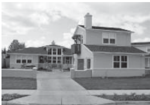
Fig. 3.1.13 This project on Old Redwood Highway in Windsor incorporates several features to minimize the impact of the garage: It features a side entry which takes the garage door off the streetscape and allows for windows along the street side; decorative garage doors are used with glass lites to add interest; a studio with balcony is added above the garage; and a low wall is features to create a semi-private parking court.
