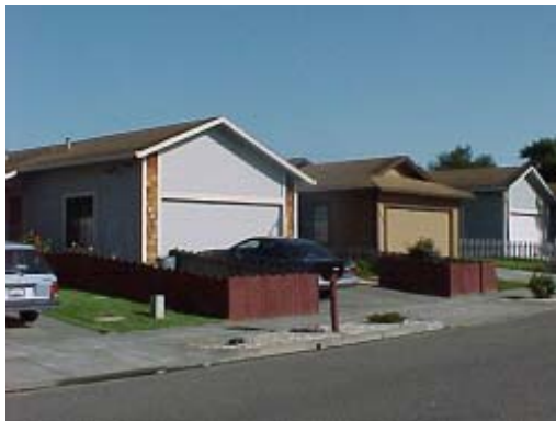
Figure 3.1.16 A garage which extends closer to the street than the front of the house as illustrated here is discouraged by the City. It moves the living portion of the home to the rear and provides little sign of habitation along the street. See Section II.F and III.G for additional information.
