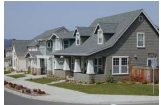
Fig. 3.1.21 This small lot subdivision in Healdsburg has variety both in the forms of the homes as well as use of materials. These three homes feature wood shingles, horizontal siding, and stucco. Additionally, the single story porch and steep pitched roof with dormers creates a two story home, but with the look of a single story. Variety of this type is encouraged.
