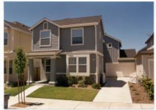
Fig. 3.1.34 Garages that are setback from the front of the home create a more neighborly streetscape.
