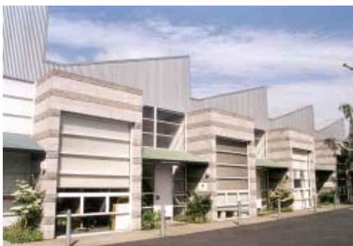
Fig. 3.4.14 This small business park in Berkeley, CA, has grouped doors and windows into a well organized visual composition. Green metal awnings are used to clearly define the entries. The use of both smooth and split-face block, combined with metal siding and a saw-toothed roof form add texture and articulation. This is a very successful design.
