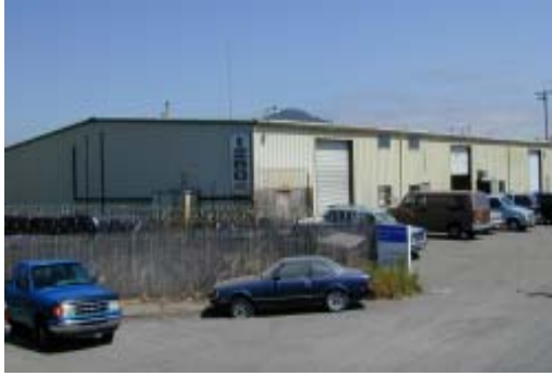
Fig. 3.4.10 Utilitarian pre-manufactured buildings such as this are discouraged.
