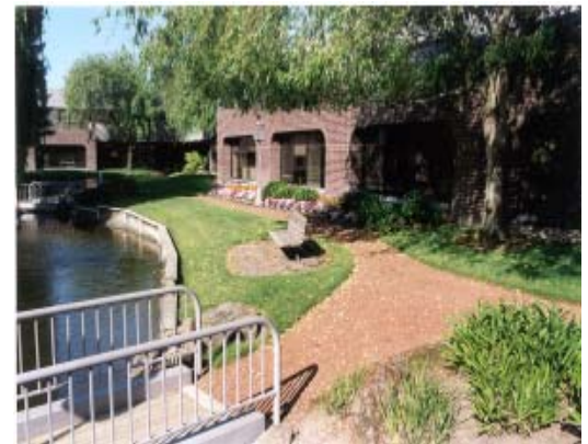
Fig. 3.4.2 The Lakes Business Park on Sebastopol Road incorporates a beautifully landscaped center court with pathways around a water feature.
