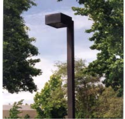
Fig. 3.4.9 A typical shielded light fixture.
