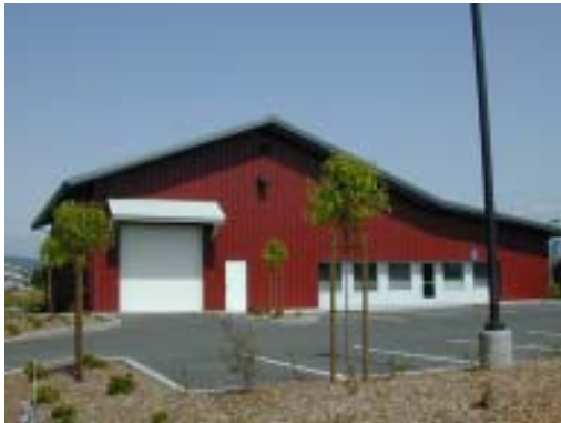
Fig. 3.4.11 Features of this building such as: roof overhang, steeper roof pitch, use of accent panels, and a sense of entry, contribute to an acceptable metal building.
