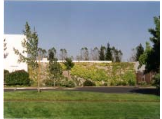
Fig. 3.4.15 This service area is effectively screened with a masonry wall that is planted with ivy.
