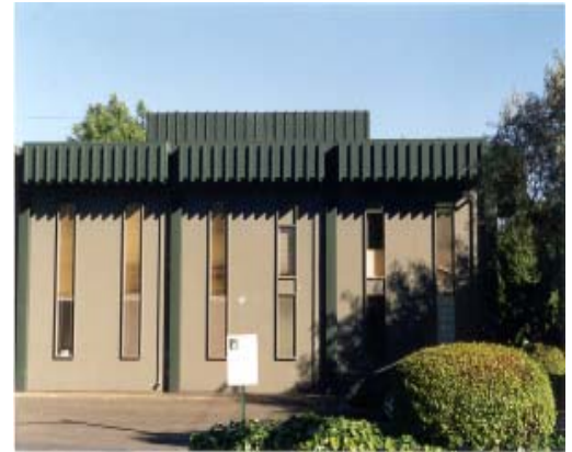
Fig. 3.4.16 This building on Second Street features an equipment screen wall that nicely picks up the detailing of the fascia.
