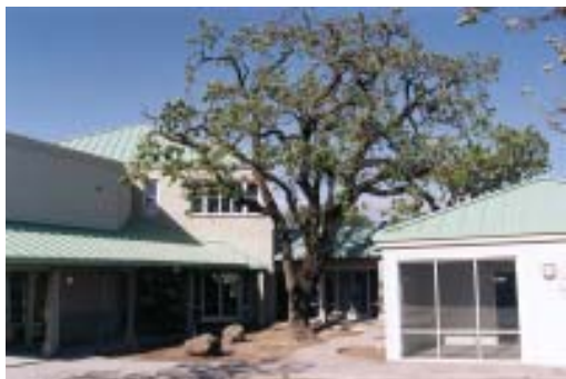
Fig. 3.4.4 This office complex on the corner of Cleveland Avenue and Jennings, incorporated the existing oak tree as a focal point of the design.
